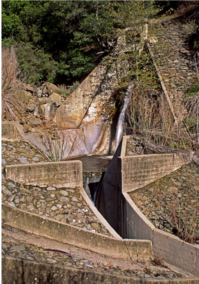
Figure 1-1. Alameda Creek Diversion Tunnel outlet.
